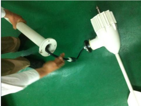
① Pass the cable through from the pole
